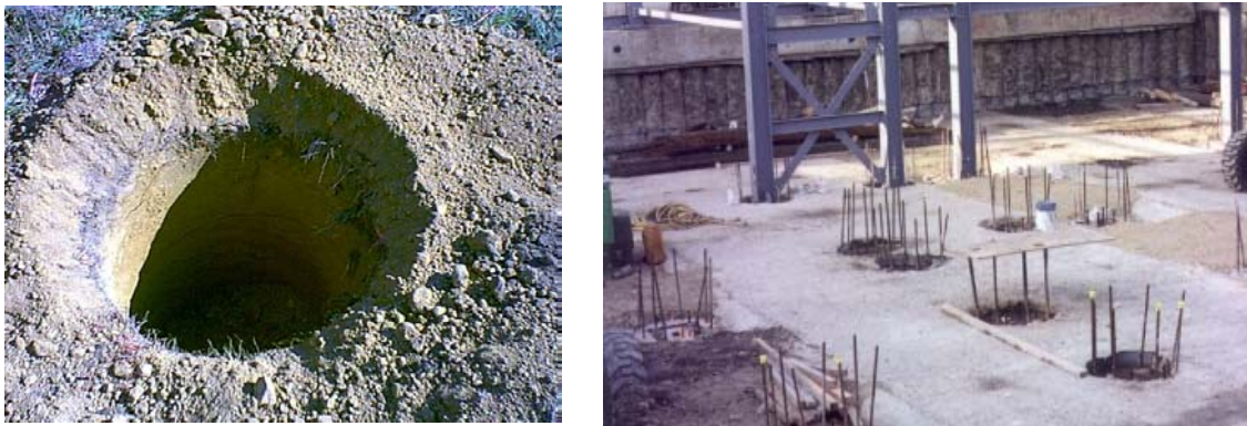
Figure 6.4: Cast-in-place pile installation process
