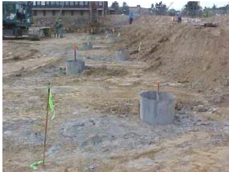
Figure 1.2: Typical cast-in-place pile layout
