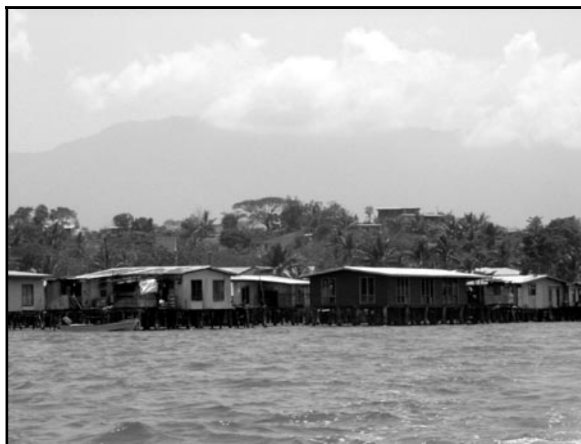
Figure 4. Houses Over the Water in Tubuseria
