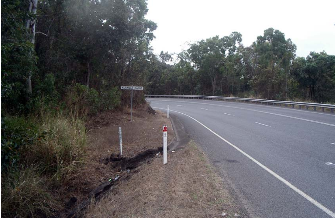
Figure 2-14: Photograph of the road surface of the Kuranda Range Road, along with a concrete drainage structure.
