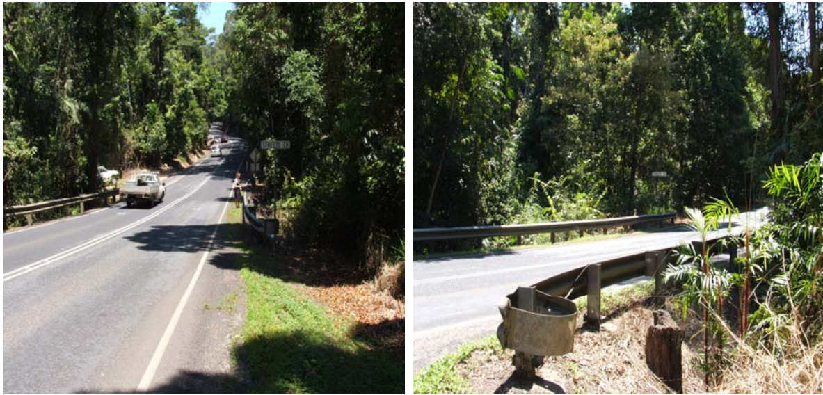
Figure 2-7: View of the existing Kuranda Range Road crossing with Streets Creek.
