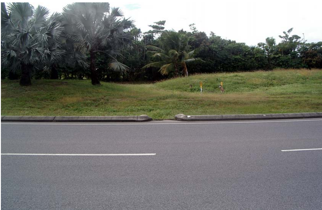
Figure 2-15: Photograph of the surface of the Captain Cook Highway roundabouts. A drainage structure common to the roundabouts is shown in the centre of the image.
