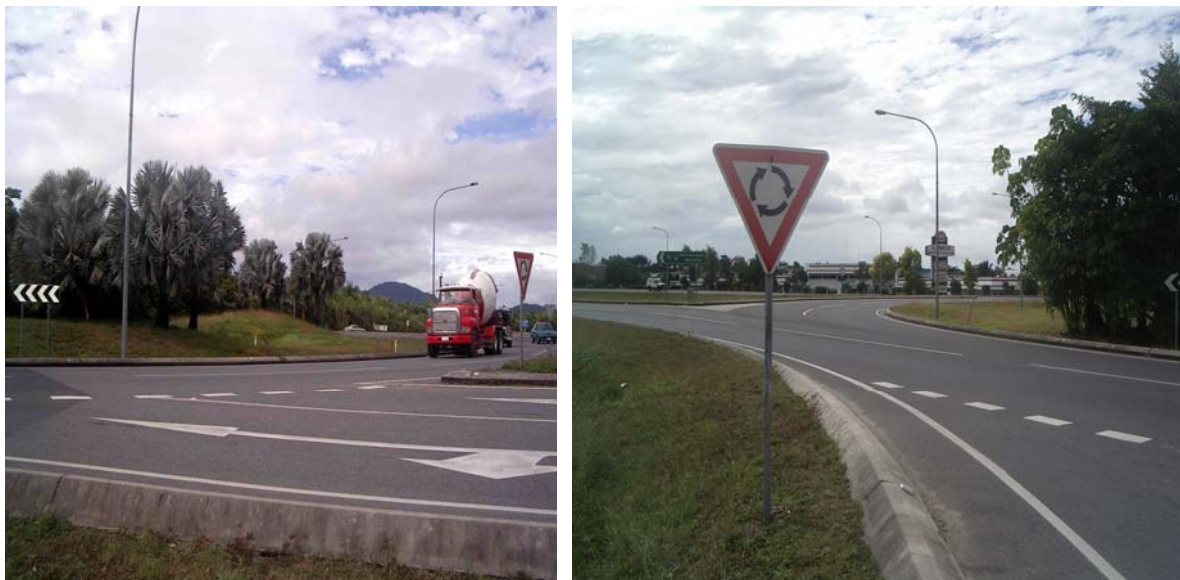
Figure 2-8: Photograph of studied roundabouts on the Captain Cook Highway.
