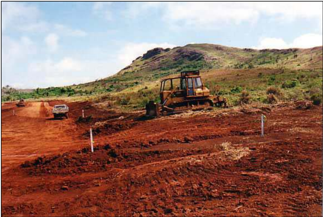
Plate 5.5 Bulldozer clearing land at Zomar, northwestern high interior of Mer
