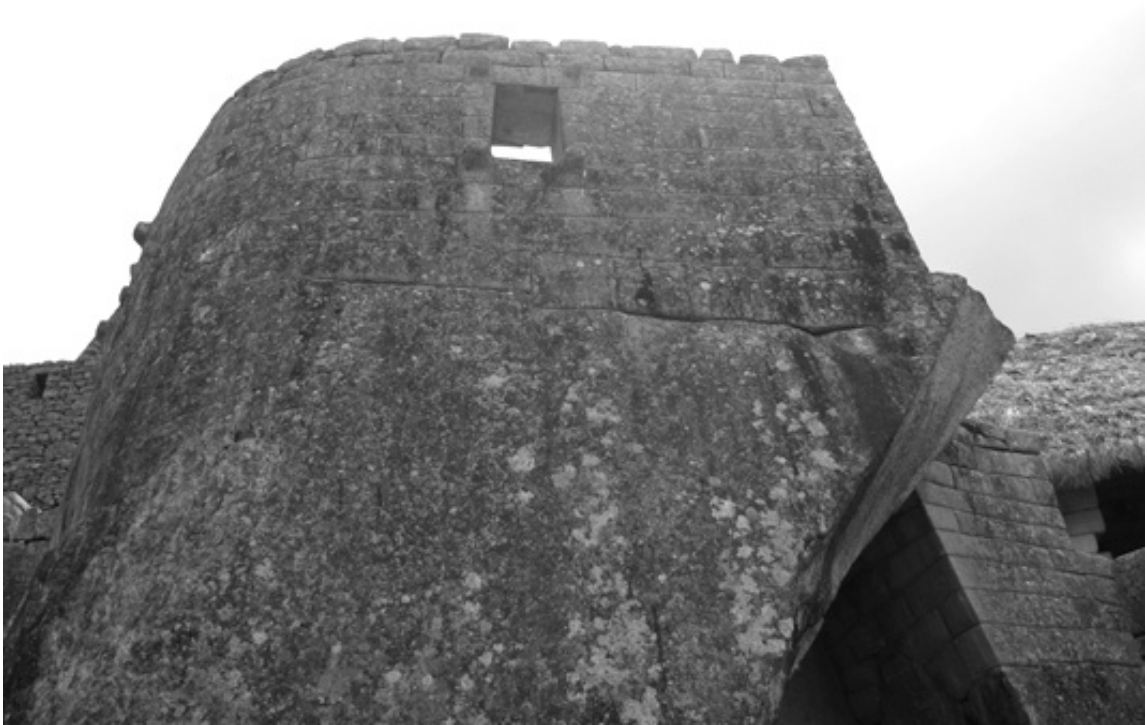
Figure 11-10: The Torreón's northeast window within its curved stone wall constructed seamlessly atop natural rock.
