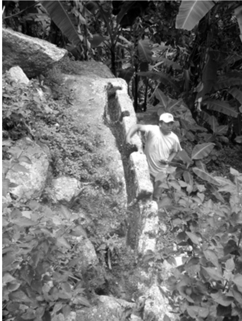
Figure 11-30: Canal with carved baffles designed to produce equal water flow in the four fountain outlets.
