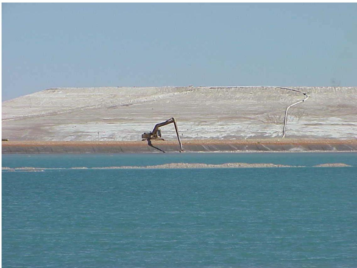
**Plate 5.1. Phosphate Hill PG Stack – Constructing Cell 4 (Cell 2 behind),
