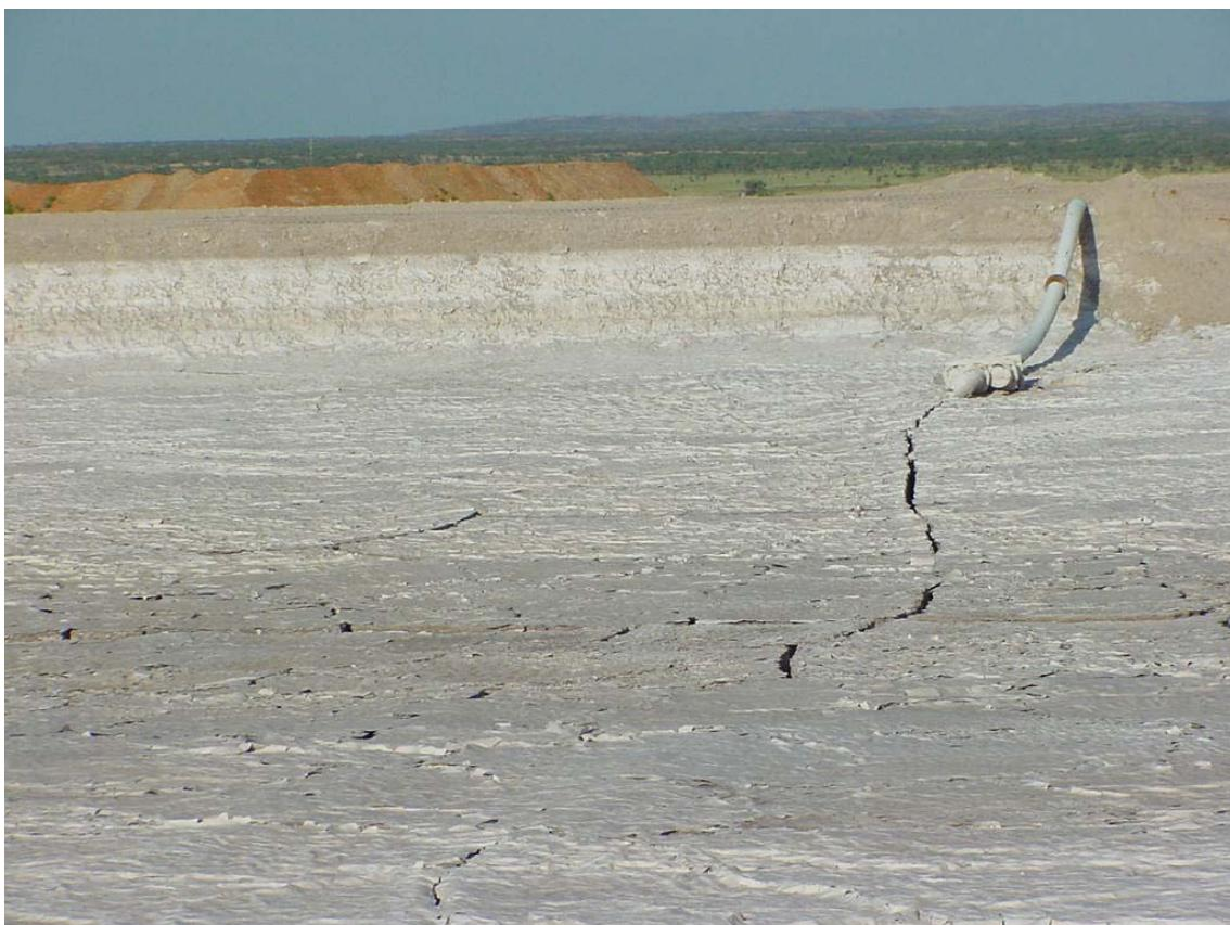
**Plate 5.3      Consolidation/shrinkage cracks developing in the top of Cells 1 and 2, Phosphate Hill, February 2004.** The cracks are tens of metres long and 10-20cm wide. The height of the stack has dropped by about 1m in approximately six months.
