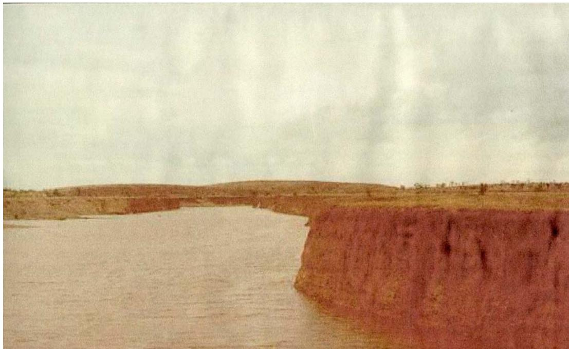
**Plate 5.2      Flooding in Galah Pit, *circa* 1975.** The water is estimated to be 8-10m deep along the right (eastern) side, becoming shallower to the left (west) and took several weeks to drain away.
