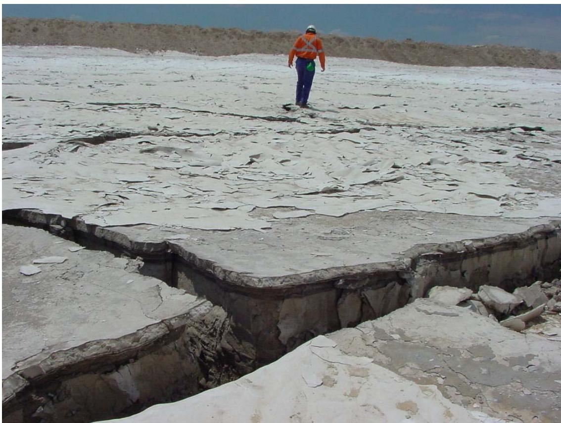
**Plate 5.4 Close-up of consolidation cracks in the centre of Plate 5.2. The surface crust that develops on the stack is clearly visible above the darker line and is 3-5cm thick.**
