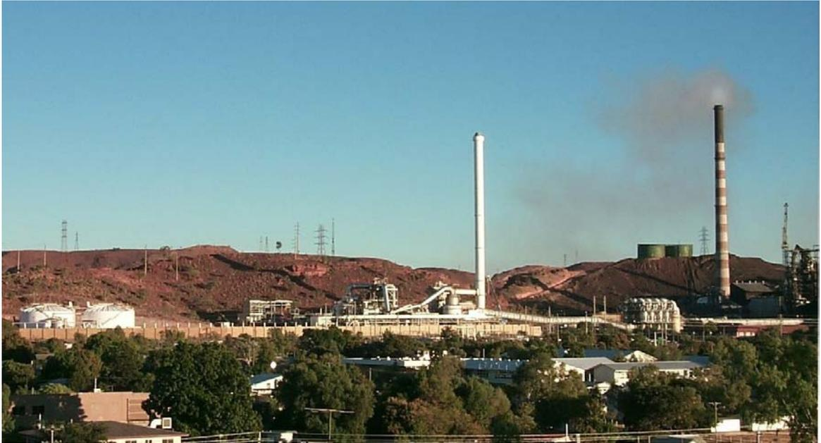
**Plate 2.12. Mt Isa sulphuric acid plant (centre) with Xstrata copper smelter to the right. Acid storage tanks and rail load-out facility on the left.**
