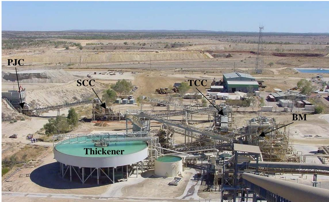
**Plate 2.8. Phosphate Hill beneficiation plant, looking east from the rail loadout hopper towards Galah North pit. The three slurry holding tanks are off the photo to the right. PJC = primary jaw crusher, SCC = secondary cone crusher, TCC = tertiary cone crusher and drum scrubber, BM = ball mill.**
