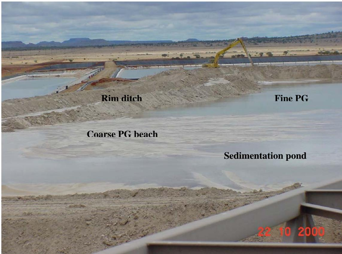
**Plate 2.14. Long-arm excavator building rim ditch, Cell 1, October 2000. Cell 2 is visible directly behind the excavator and the return surge ditch is visible to the left.**
