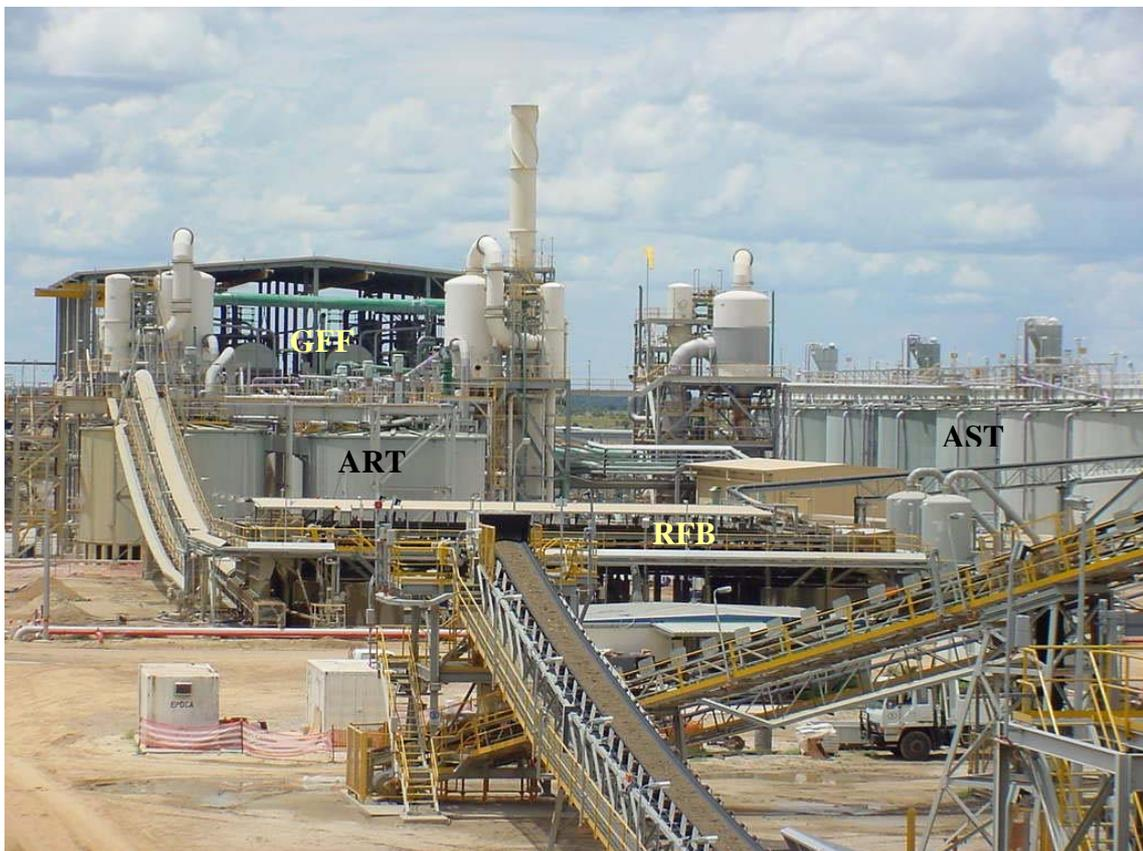
**Plate 2.9. Phosphate Hill PAP looking north over beneficiation tertiary crusher. RFB = rock slurry filtration belts, ART = acid reactor tanks, GFF = gypsum filter belt floors, AST = acid storage tanks.**
