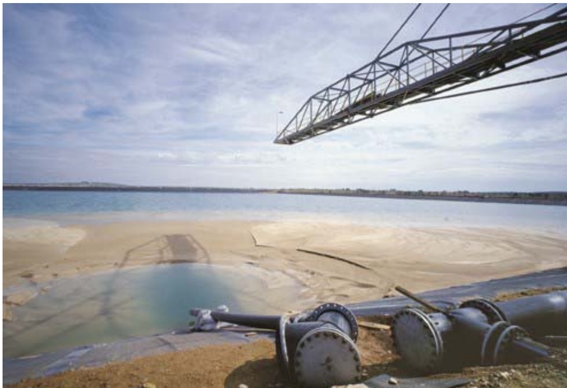
Plate 1.2. Phosphate Hill PG Stack (Cells 1 & 2)
