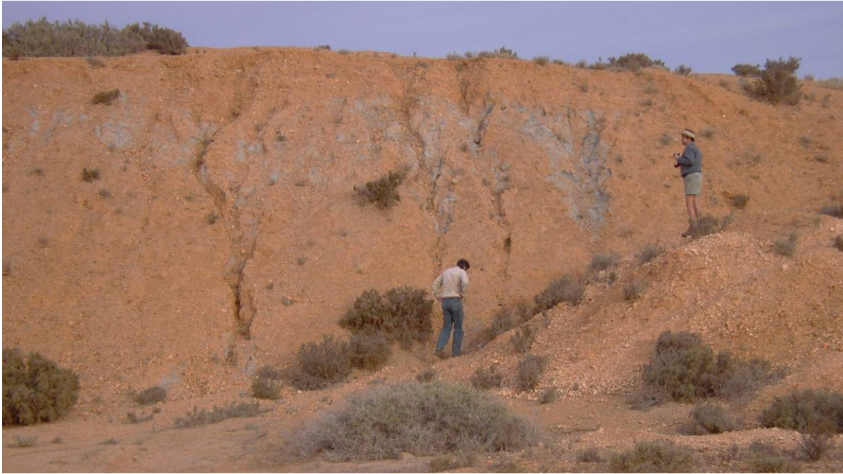
Figure 3: Rill erosion of the soil capped tailings storage facility, Radium Hill, South Australia (height of facility approximately 6 m). The soil capping is being removed, resulting in the exposure of radioactive tailings in rills.
