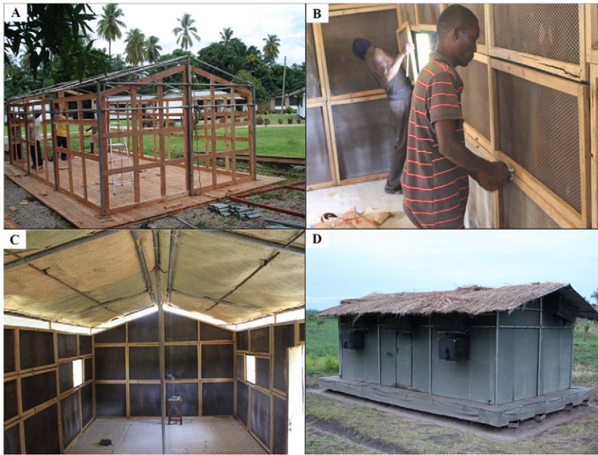
Figure 3. Pictorial representations of selected steps in the construction of the Ifakara experimental huts. Panel A shows the main framework of the Ifakara experimental huts under construction at the workshop. Panel B shows technicians fitting the wall panels, (which are made of chicken wire on wooden frames), onto the inside walls of the Ifakara experimental huts. Panel C shows the inside surfaces of the huts after fitting the chicken wire wall panels and also the palm woven ( mikeka ) ceiling on the underside of the roof, but before the inside walls are covered with mud, and Panel D shows a completed and functional Ifakara experimental hut, fitted with interception traps on windows and eave spaces. It should be noted that the overall shape and dimensions are set to match the typical local houses, shown in Figure 1. The hut is suspended on water-filled metal bowls to prevent predator ants, which would otherwise prey on the trapped mosquitoes. doi:10.1371/journal.pone.0030967.g003
