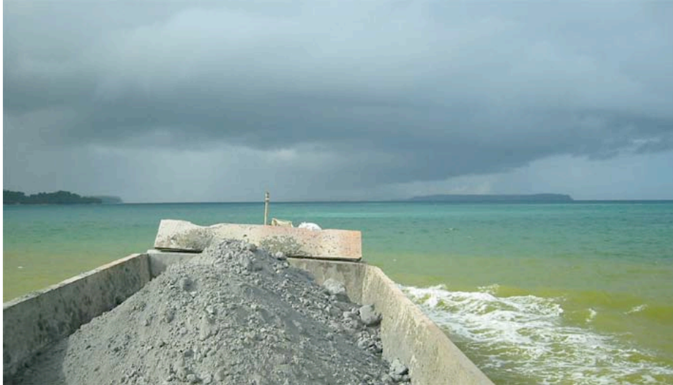
Plate 2. Photo of waste rock on split-hopper barge at dumping site (note the brown colour of the sediment plume in surrounding waters from the previous barge-load)
