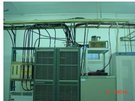
Figure 5.37 - D6 operational in Wunongchang base station
