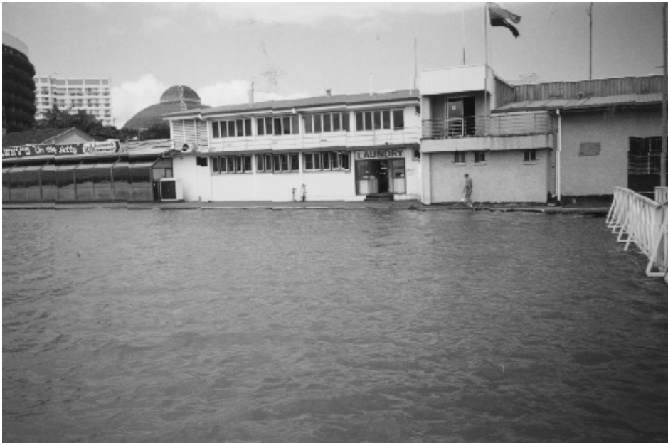
Figure 4.5 Cairns building near foreshore during spring tide
