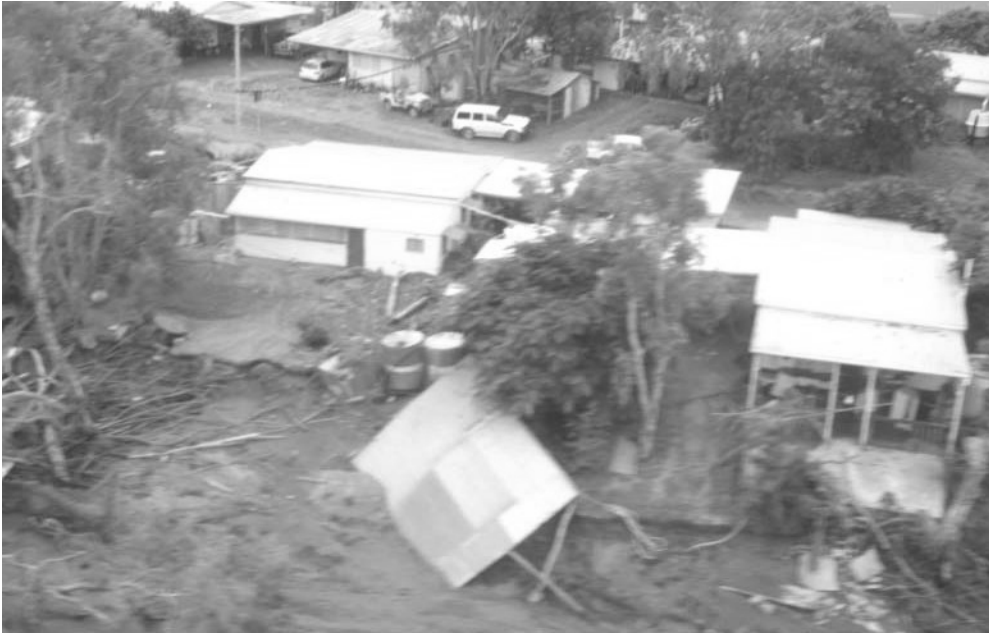
Figure 3.2 Damage to the Black River settlement in Thuringowa following floods in 1998.
