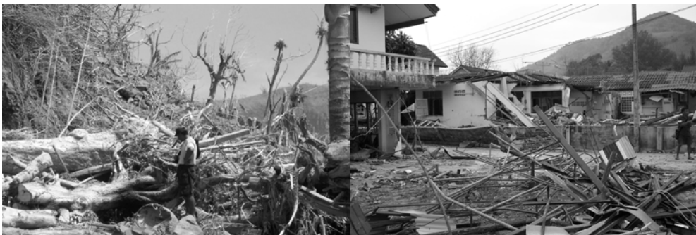
Figure 3.3 Storm surge damage at Tikopia Solomon Islands, left, and tsunami damage at Phuket Thailand, right.
