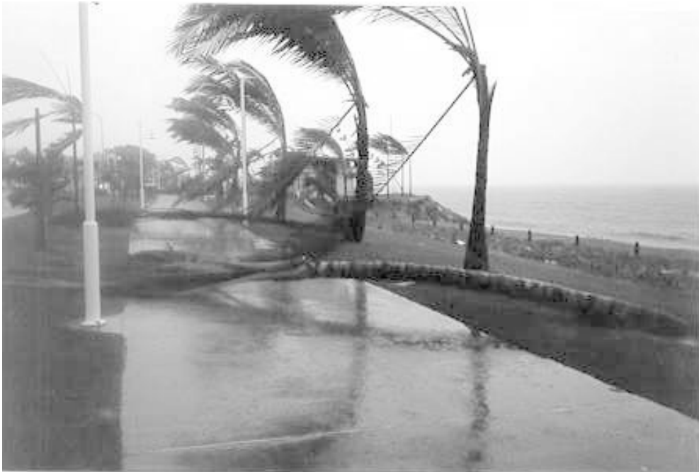
Figure 3.1 Cyclone Tessi damaged Townsville's Strand in 2000, just after reconstruction had been completed following severe damage caused in 1998 floods.
