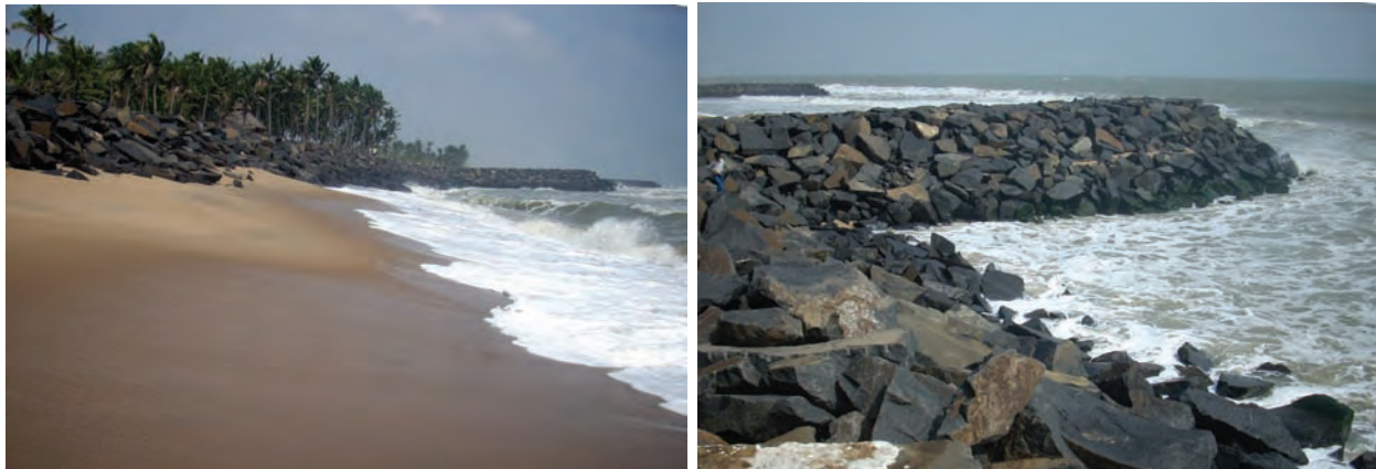
(a) A sand deficient beach.
