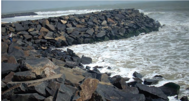
Figure 2.14: Groynes constructed along and to the North of the Pondicherry coast.
