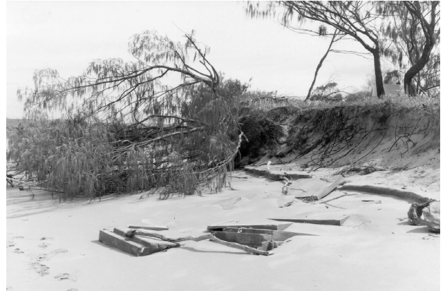
Figure 7. Creek bank erosion, north bank of Middle creek, facing northwest (Photograph: S. Ulm).
