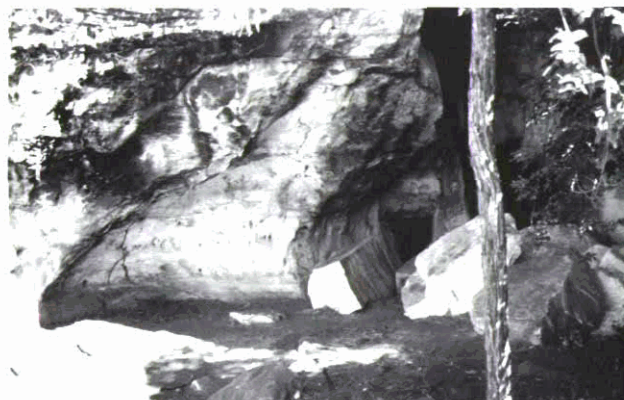
Figure 1. General view of Roof Fall Cave (Photograph: T. Eales).
