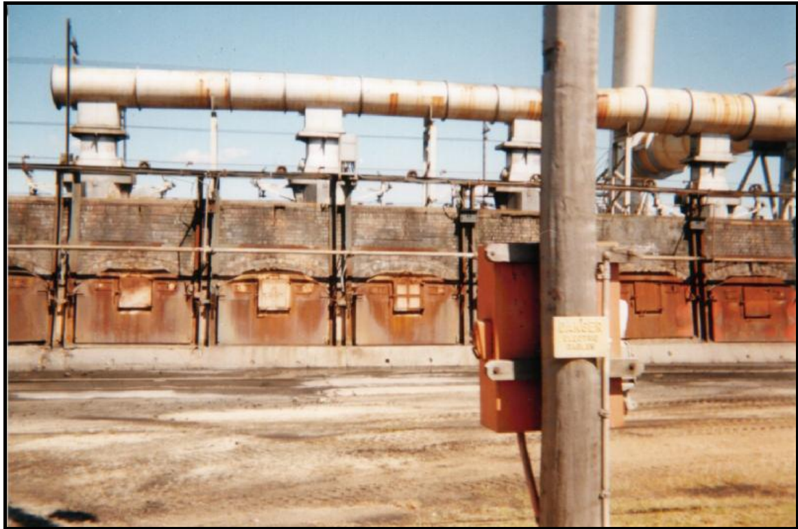
Figure 6.1. Bowen Coke Works.
