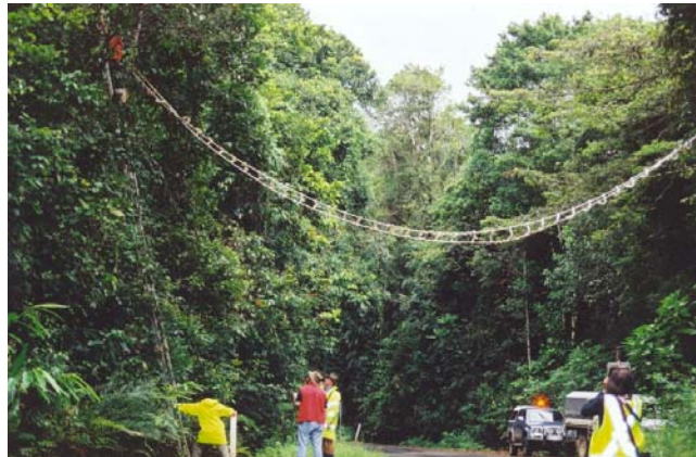
Figure 4.4 Canopy bridge being installed over the Old Palmerston Highway, April 2001 (Photo: Sue Frankcombe)
