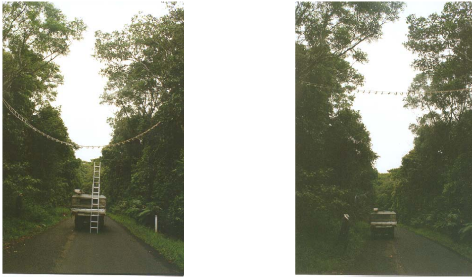
Figure 5.17a, left, Old Palmerston Highway bridge after being vandalized in early December 2001 (ht. 4.75 m) and b, right, Correct height of bridge (ht. 7.5 m)
