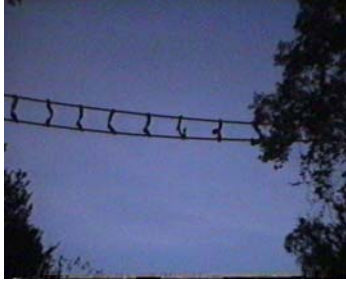
Old Palmerston Highway bridge
