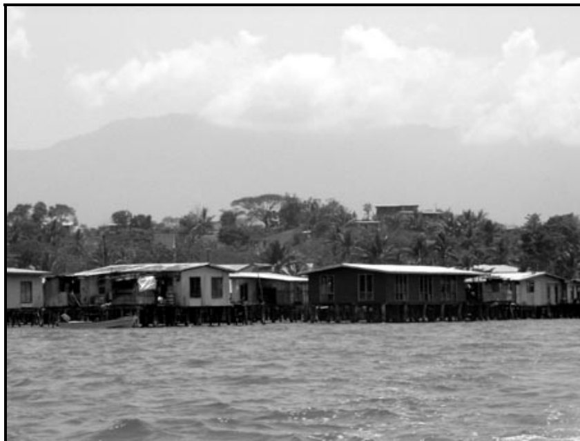
Figure 4. Houses Over the Water in Tubuseria
