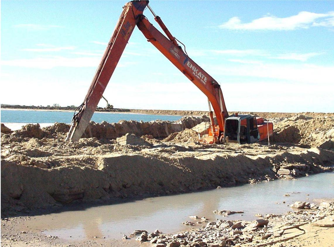
**Plate 4.12** 30 tonne excavator sunk into perimeter dyke PG, Cell 1, Phosphate Hill, April 2000. The excavator body sank until it was floating on the base of the cabin and the bucket was also completely submerged in liquefied PG.
