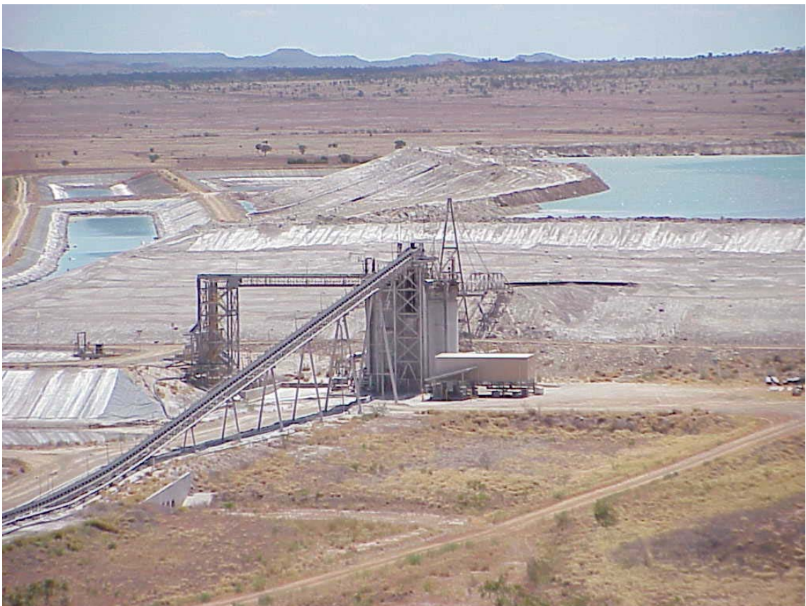
Plate 3.1. Phosphate Hill PG Stack (Cells 1 and 2) and Re-slurry Tank April 2002
